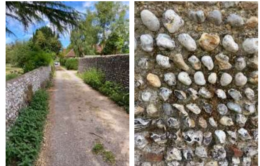
Fig 22: Historic flint walls
