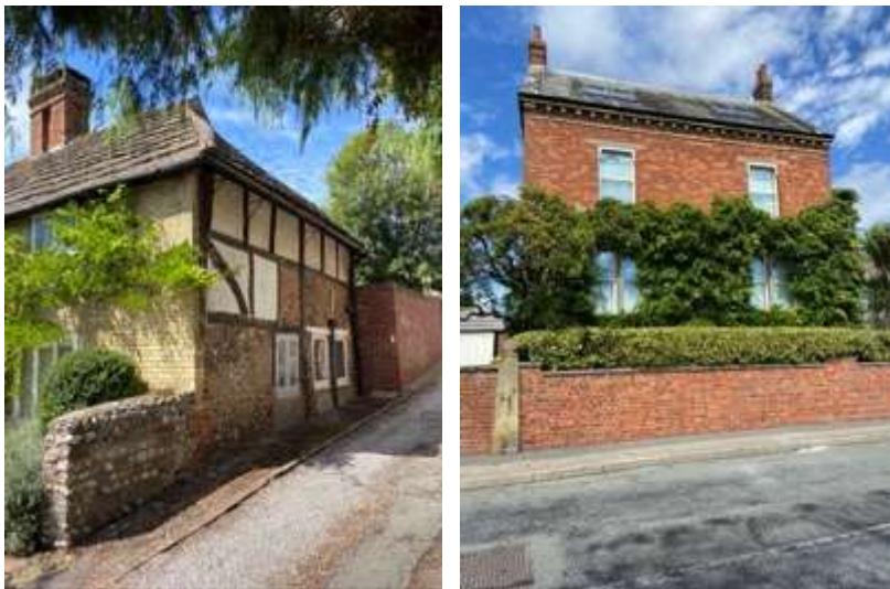
Fig 20: Use of brick in the conservation area, Horsham slab to roof of Grant's Manor
