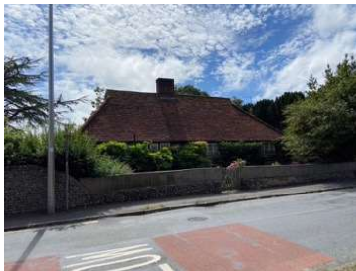
Fig 24: Close-boarded fence over reduced flint wall
